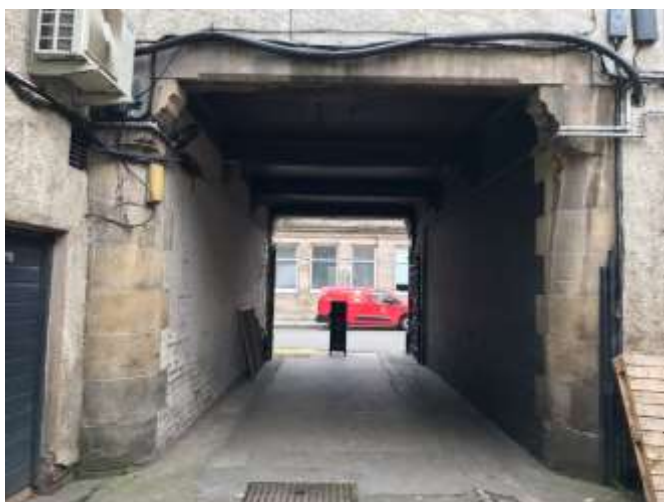
Pend running below the property to provide access to the rear
