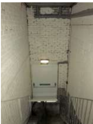
Former escape stair (access stair)
