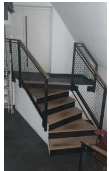
Stair to front door
