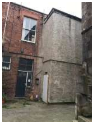
Door to access stair-ground level
