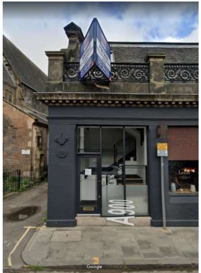
Main Entrance with secure entry phone
